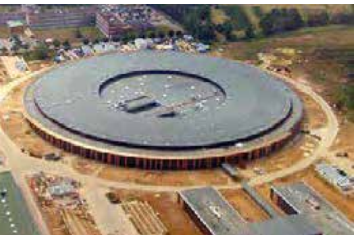
Fig. 2.6: The SOLEIL synchrotron Saint-Aubin, France.
