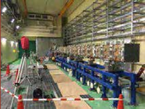
Fig. 5.8: The linear IFMIF prototype accelerator, being installed in Rokkasho, Japan.
