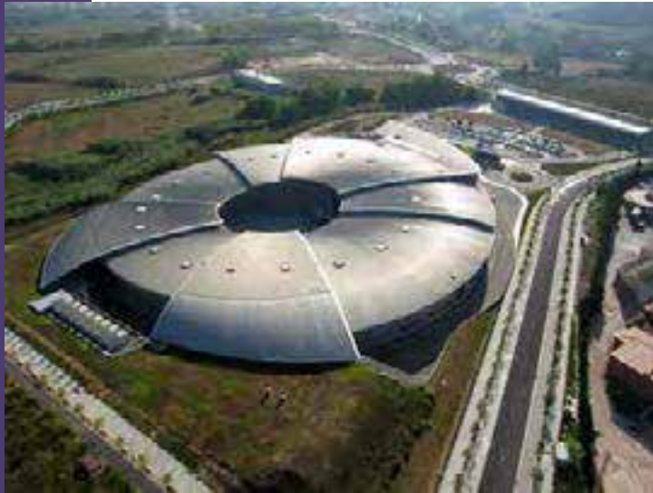
Fig. 7.3: An aerial view of the ALBA light source near Barcelona, Spain.
